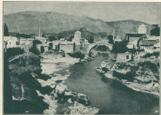
Narentabrücke in Mostar.
