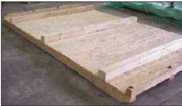
Provision of the platform with support timbers placed on top
