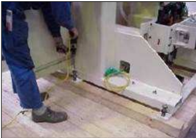
The holes for the fastening bolts and the corresponding bolt holes in the support timbers are drilled.
