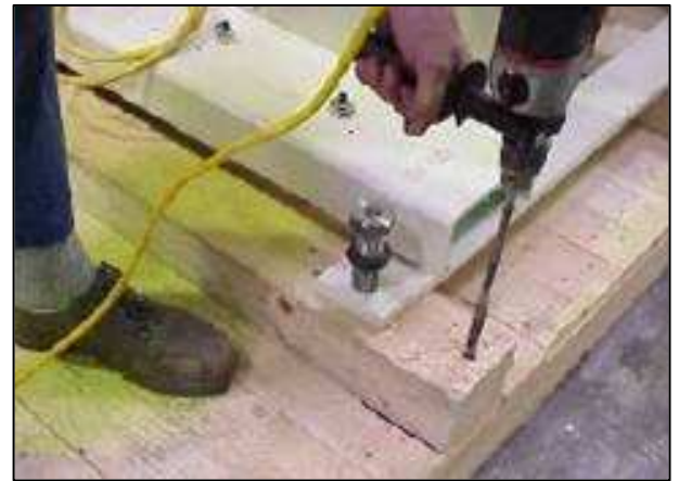
The holes for the fastening bolts and the corresponding bolt holes in the support timbers are drilled.
