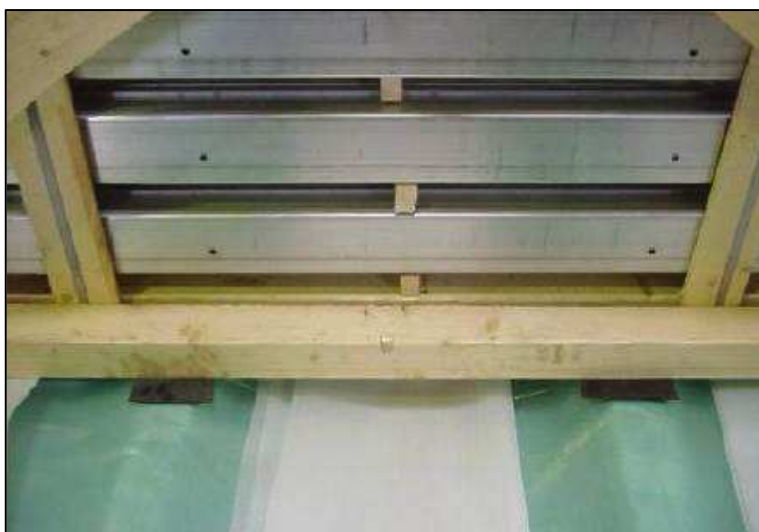
Nail down the stop blocks.
