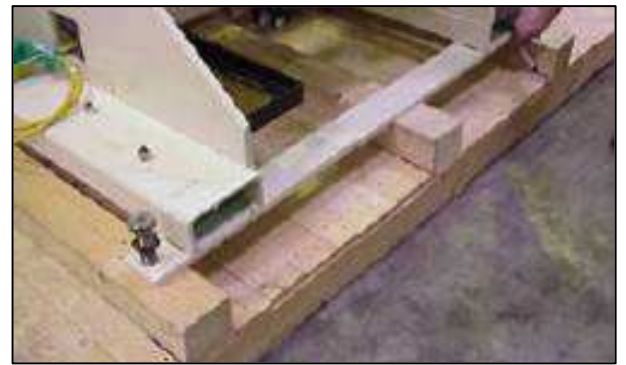
The machine has been positioned and the locations of the support timbers are marked.
