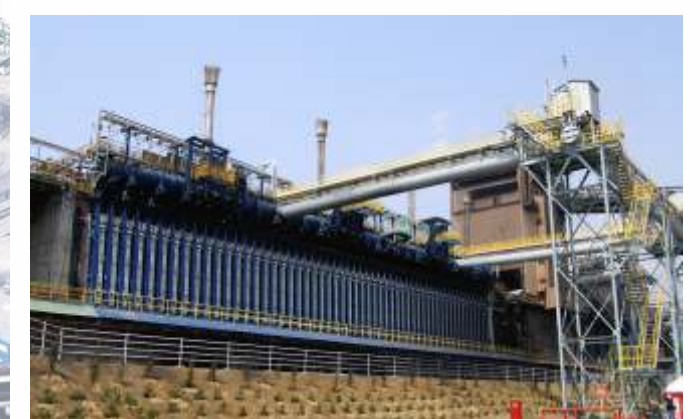
Coke Oven Battery
