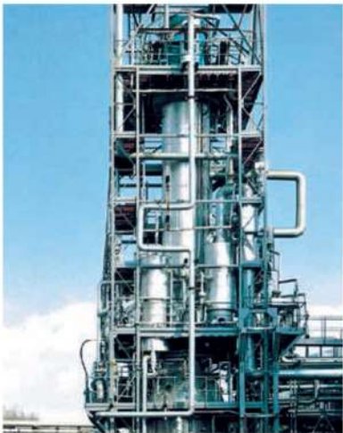
350 mtpd Methanol plant (grade AA) using innovative synthesis gas generation from waste products such as: clarifier sludge, used light and heavy oil, rubber waste, contaminated wood, and shredded material from recycling plants of motor vehicles. SVZ GmbH, Schwarze Pumpe, Germany
