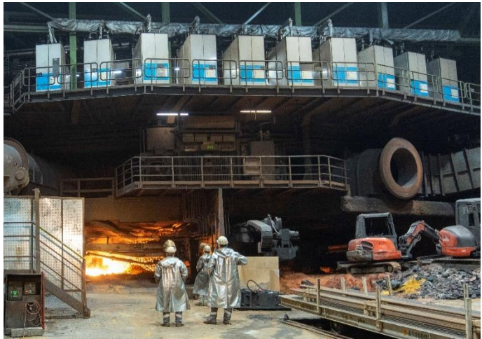
Image 1: View from cast house floor at Schwelgern BF1 where SIP Technology is installed
