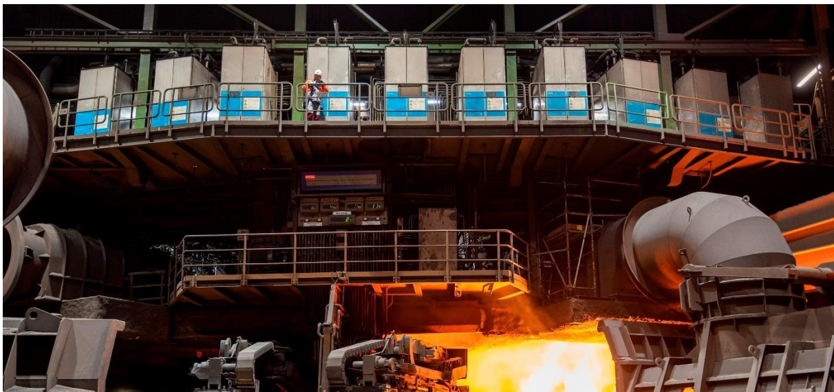
Image 1: View from cast house floor at Schwelgern BF1 where SIP Technology is installed
