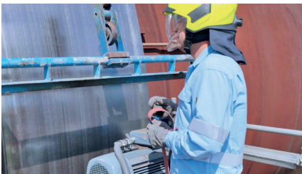
polgrind® slide ring and tyre grinding
