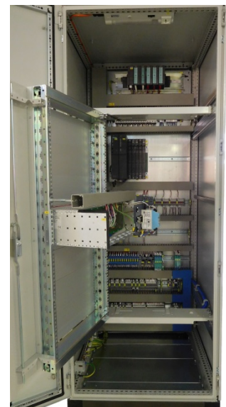
Reactor controller with opened cabinet door Inner workings with opened swing frame
