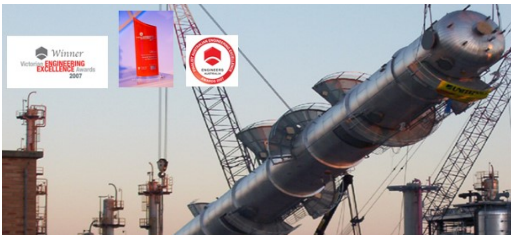
Module being transported and lifted into position at Altona Refinery.
