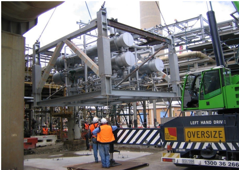
Module being transported and lifted into position at Altona Refinery.
