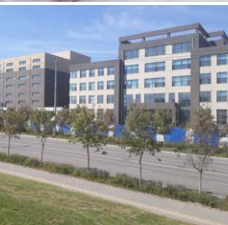
PLA plant for COFCO | PLA Anlage COFCO
