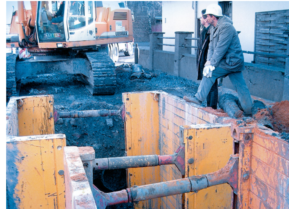
KS 100 Eck: Simple, cost-effective shoring for circular and masonry manholes.
