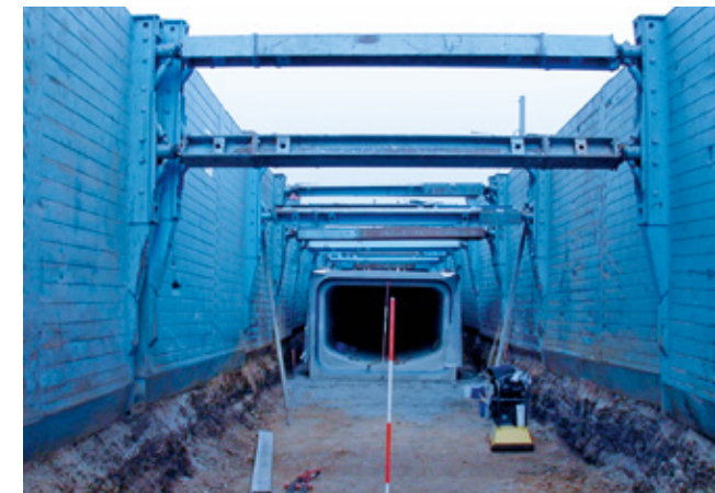
Drag box – for shoring projects carried out in open and mainly unbuilt terrain.
