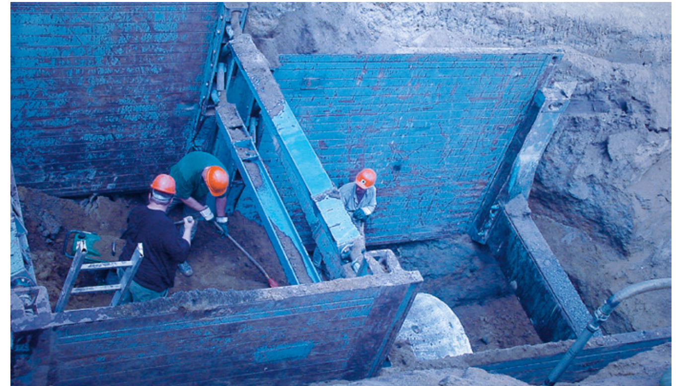
Drag box – for shoring projects carried out in open and mainly unbuilt terrain.
