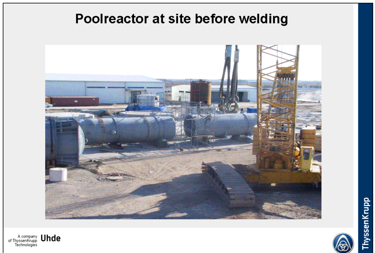
Figure 5: Tecen pool reactor in two pieces before welding
