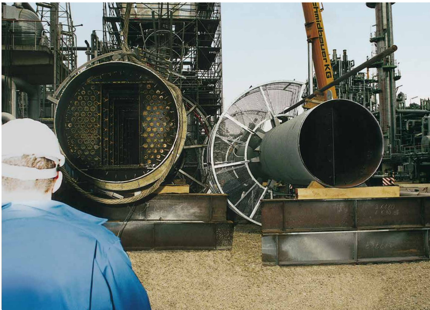
New divided wall section before installation of packings
