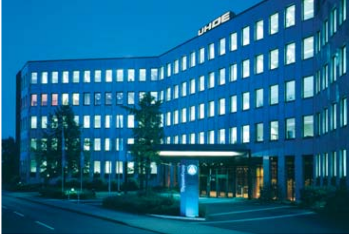
Head Office and engineering offices of Uhde GmbH in Dortmund, Germany
