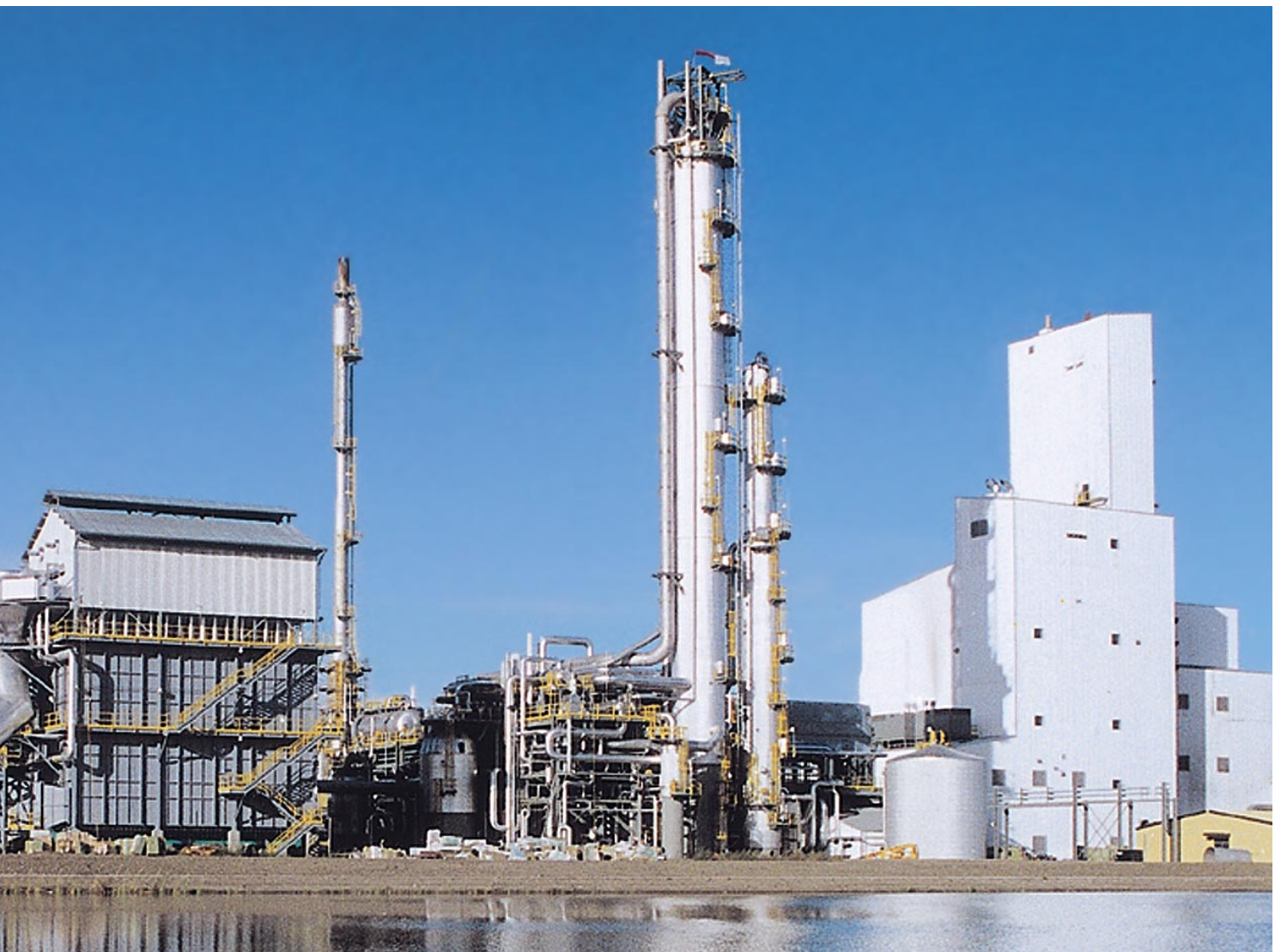
| Saskferco ammonia-urea complex, Canada
