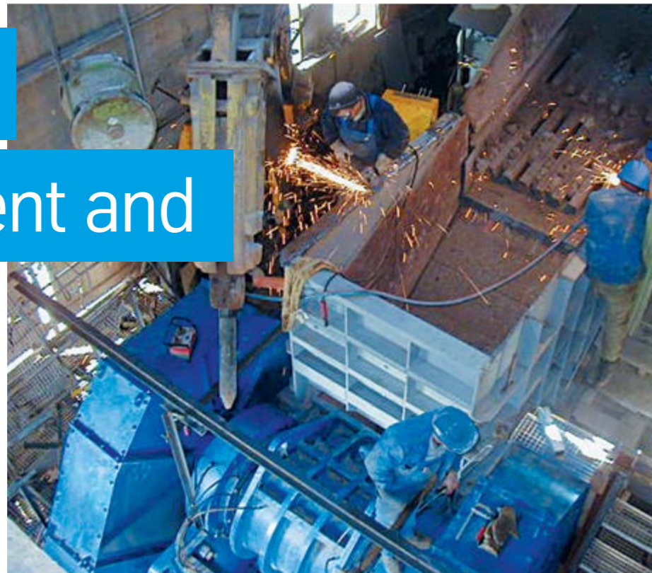
Installing a heavy-duty single-toggle jaw crusher to modernize a quarry
