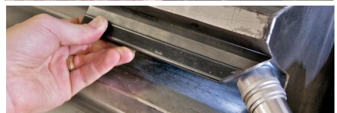
Fig. 1: Measurements at planetary gear units with the vibration measuring device
