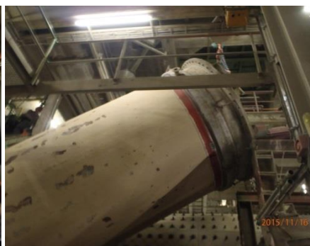
Powder cooler during disassembly and assembly phase
