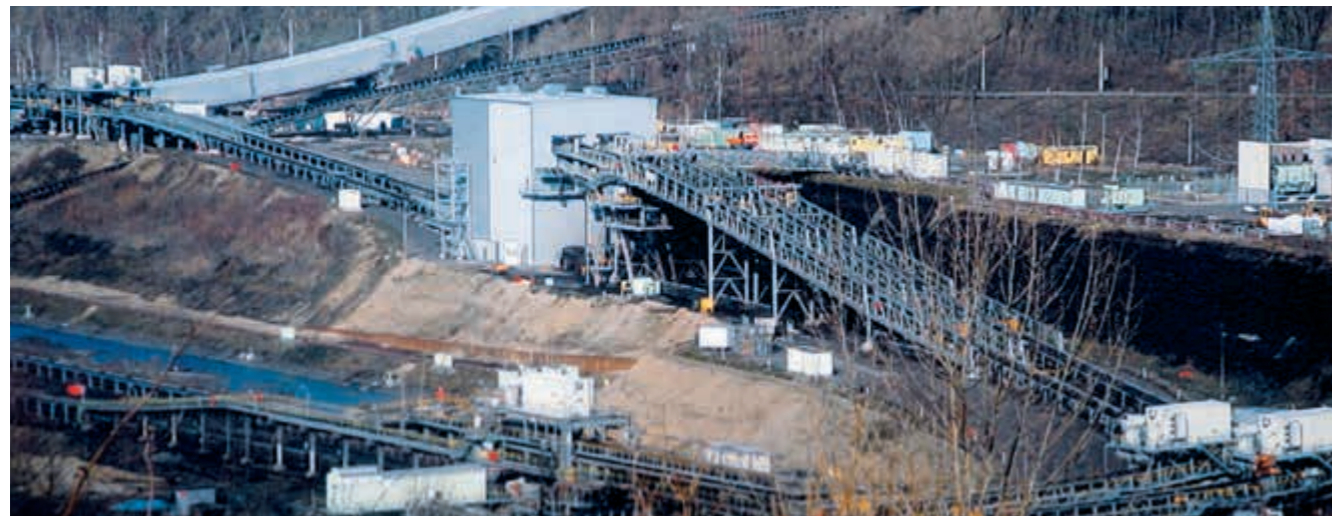
Lignite processing plant built by thyssenkrupp Industrial Solutions with four RollSizers, DRS 660 x 3700 SideSizers, in operation.
