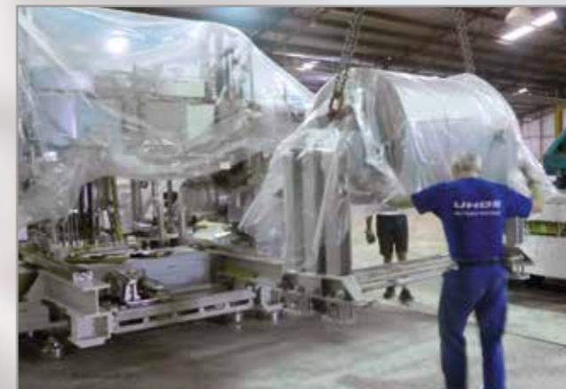
Installation of the plant by trained staff
