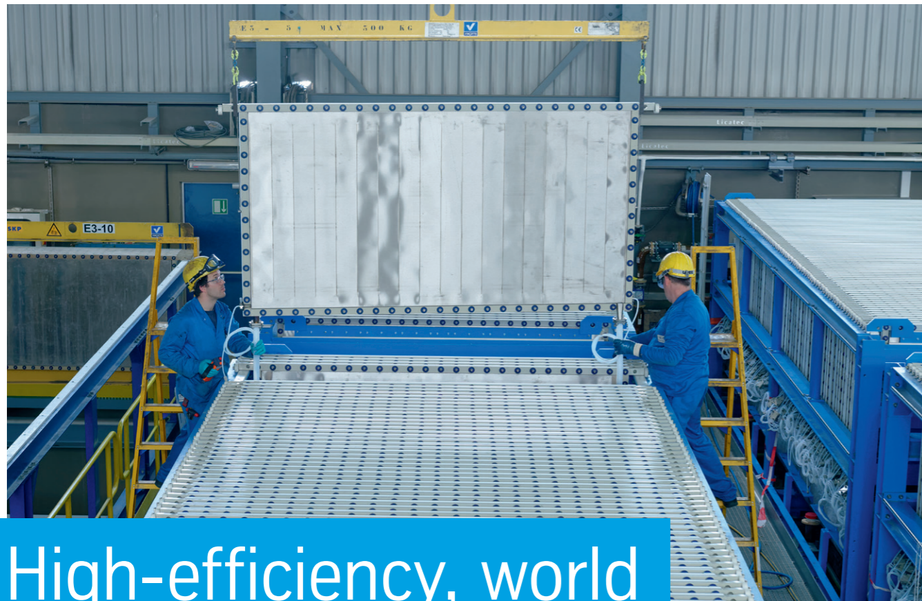
Picture: electrolysis plant during construction.
