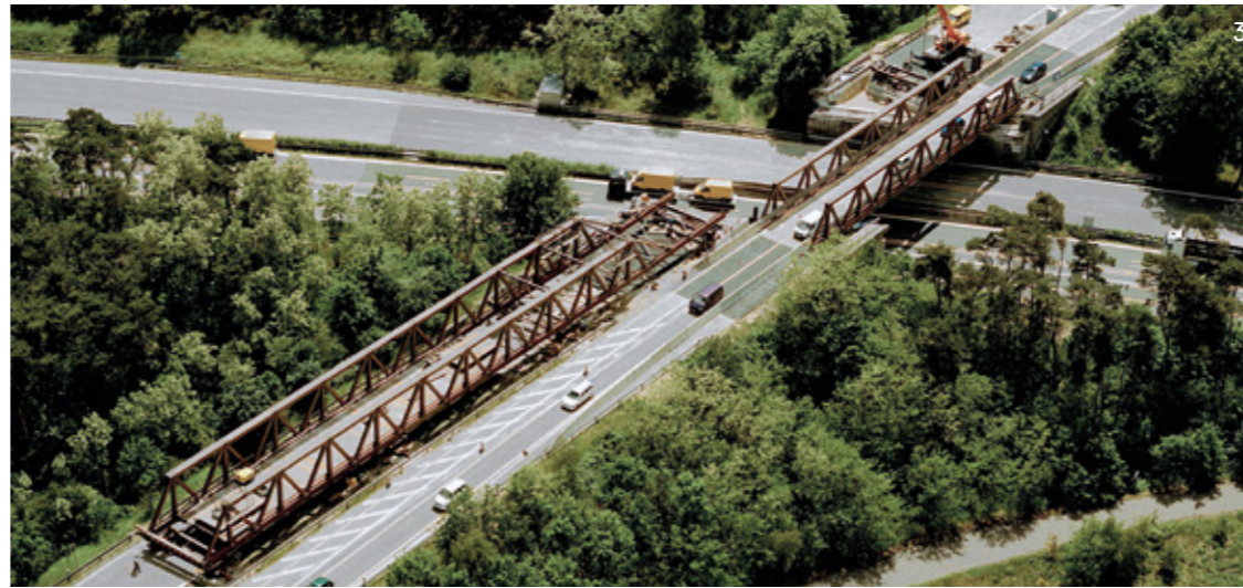
3 Temporary bridge carrying the A115 over the A10, Nuthetal freeway junction.
