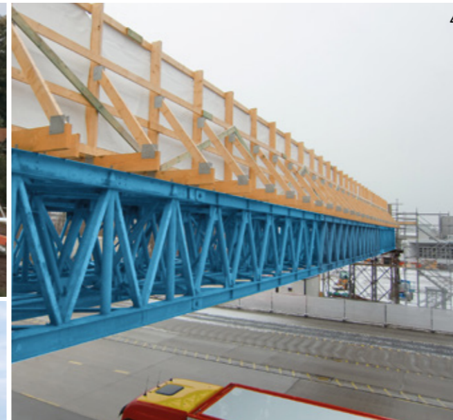
4 Pedestrian bridge over a vehicle manufacturer's test track.
