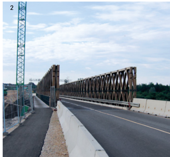
2 Temporary bridge with a single-side cycle lane and sidewalk over the Main River at Breitengüßsbach.
