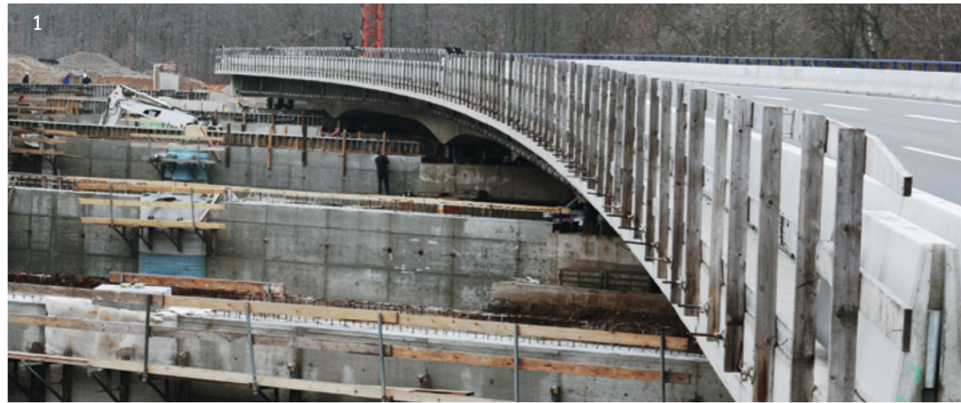
1 Reconstruction of Braunschweig southwest freeway junction.
