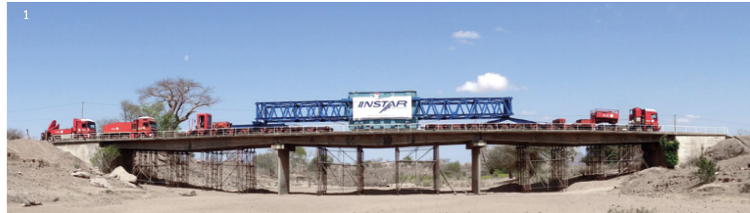
1 Transportation of transformers in Mozambique.
