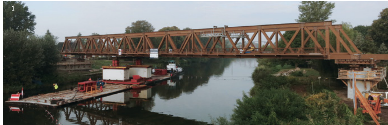
1 Construction of the new Marquardt road bridge over the Sacrow-Paretzer Canal.
