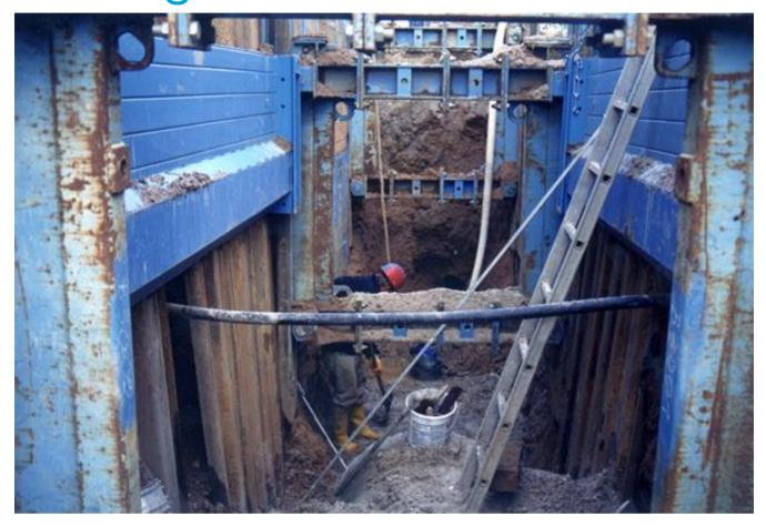
In urban areas, trench sections crossed by numerous pipes and cables are commonplace. Using large-area shoring systems is then out of the question. The solution is inner-city linear shoring that combines the piling frame element for guiding sheet piles with the components of the linear shoring system.
