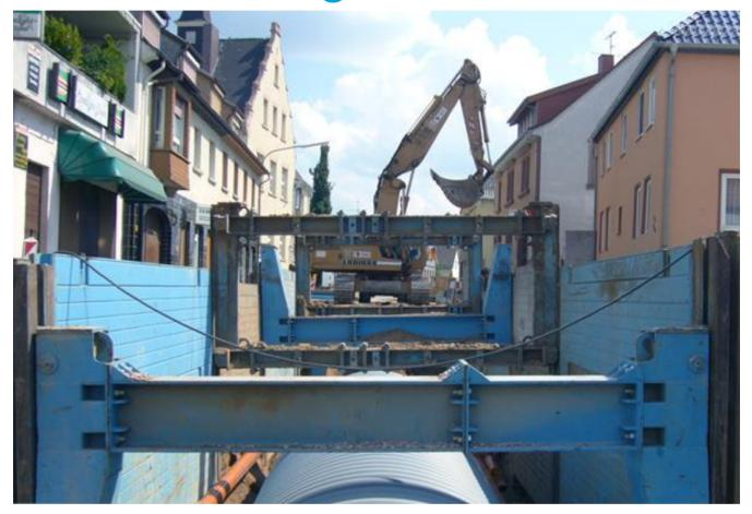
Linear shoring is suitable for casting concrete in-situ place and can be flexibly adapted to any construction project. The ground outside the trench remains largely unaffected, and buildings and traffic flow are not impaired — a level of performance that was long-considered unattainable.
