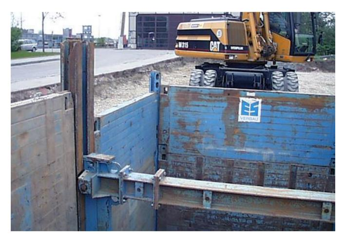
Corner rail shoring is a special shoring solution, suitable among other things for work on manholes. When used as manhole shoring, it usually consists of four slide-rail panels and four corner rail beams.
