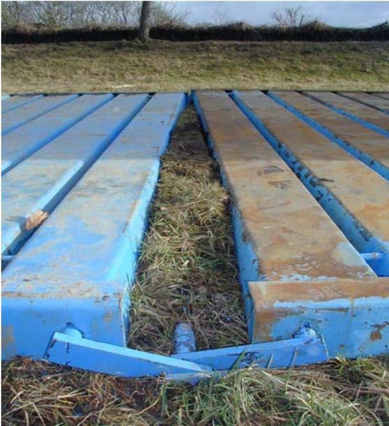
With two locking straps and one locking bolt the creation of a curved radius of about 40 m is possible.
