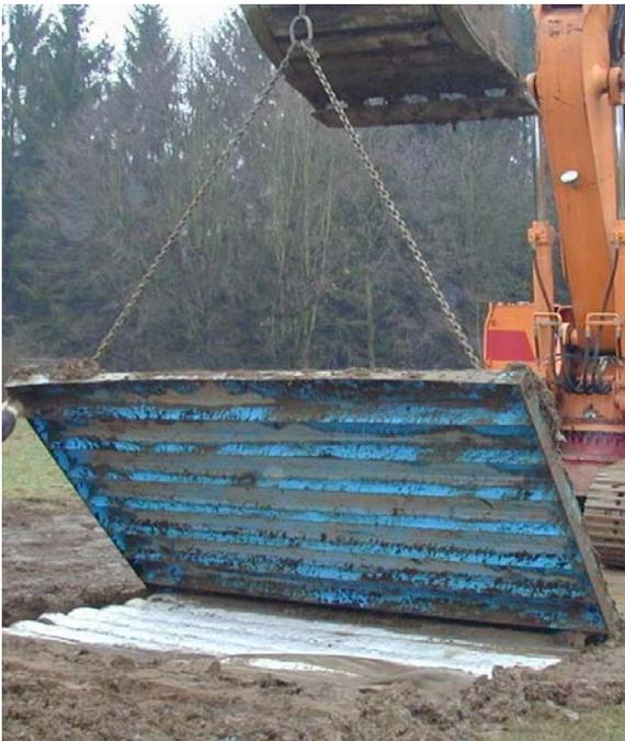
For re-mounting and separation of the panels, lifting may only occur at the designed lifting points (round bolts on top) with 2 hooks at the one side (min. 13 mm chain, 16 mm possible, chains supplied by contractor).
